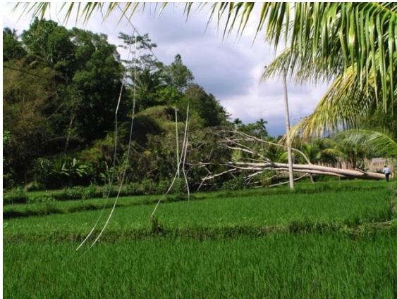
Figure 3: Example of a storm damaged distribution line. A tree has fallen onto the MV transmission line.
