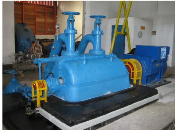
Figure 27: Adjustable spear valve on a pelton turbine.
