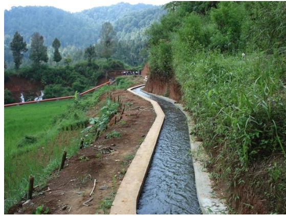
Figure 32: Stone masonry headrace channel in operation.
