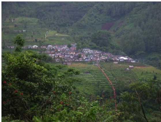
Figure 7: Typical rural village in a mountainous area supplied with a stand-alone MHP project.
