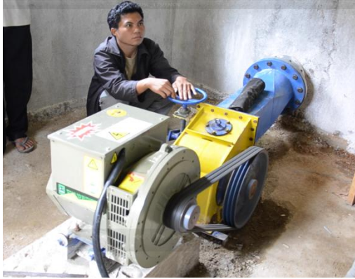
Figure 34: V belt step-up transmission with pulleys fixed directly on generator / turbine shafts.
