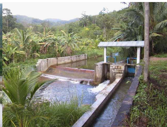
Figure 17: Conventional weir and intake structure.
