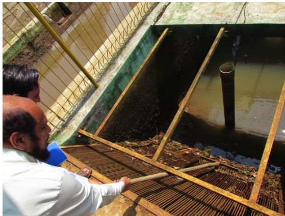
Figure 91: Cleaning the trash rack whilst the forebay is empty
