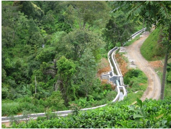
Figure 31: Ariel view of stone masonry headrace channel with spillway and pipe bridge visible.
