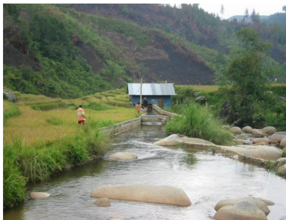
Figure 16: A semi natural intake structure whereby the stream flow is diverted to the powerhouse without construction of a weir.
