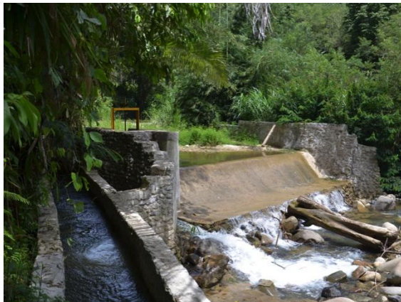
Figure 21: Typical stone masonry weir and intake structure.
