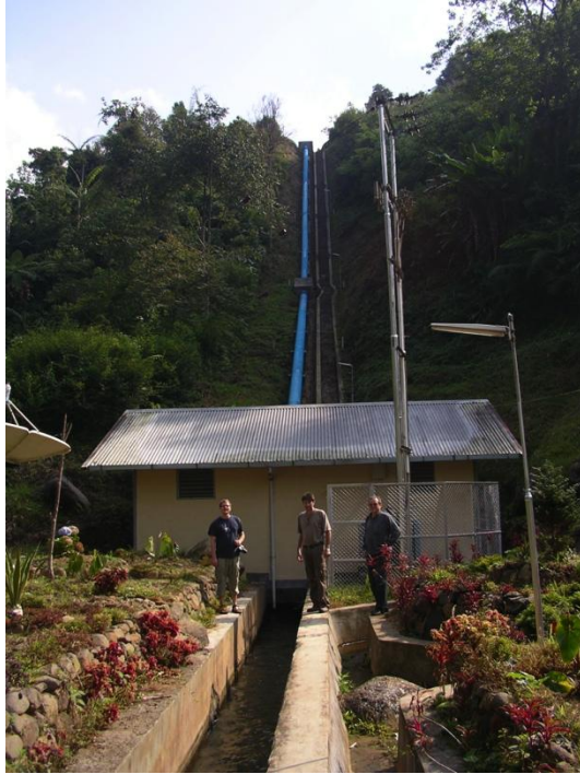
Figure 53: View from riverbank of penstock, powerhouse and straight tailrace returning the water to its original source.
