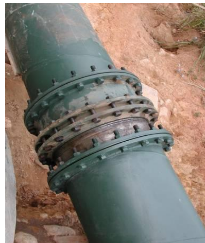
Figure 48: The most common type of joint is the mechanical sliding type pictured here.
