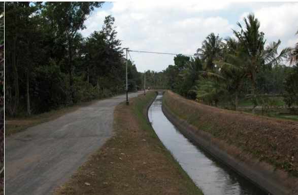
Figure 30: Trapezium shaped concrete lined channel.
