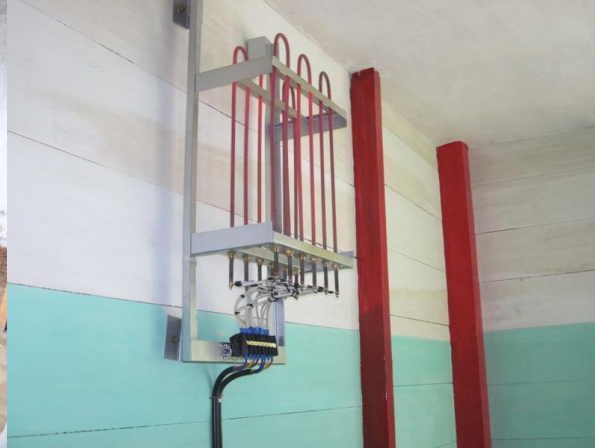
Figure 98: Once the ballast has been loaded sufficiently, consumer load can be connected.
