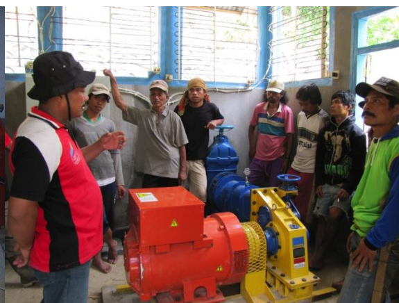
Figure 68: Shaft-to-shaft direct drive arrangement. This scheme does not have a flywheel as it is controlled with an ELC.
