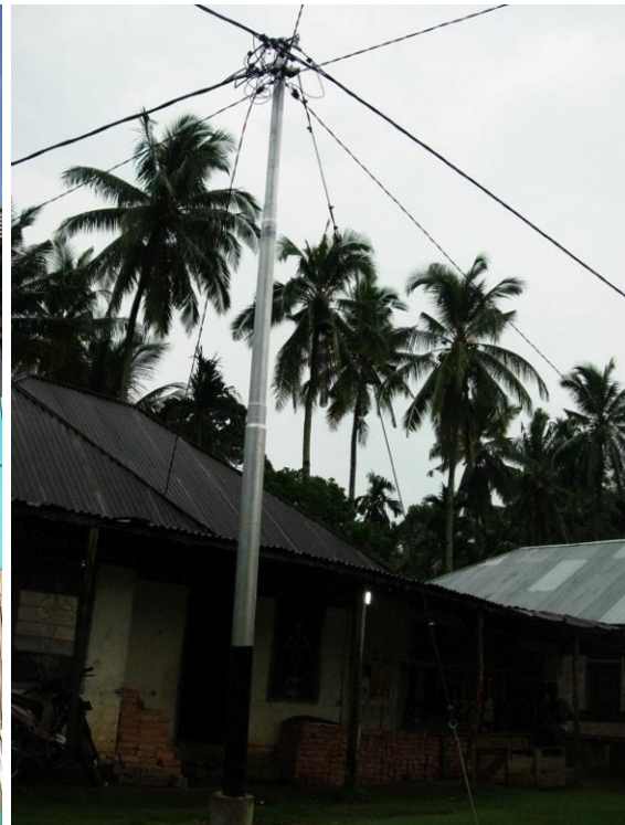
Figure 82: Example of a 2 section steel cable pole.
