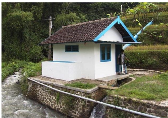
Figure 20: Powerhouse of a 15kW MHP.
