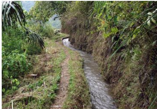
Figure 29: Low cost unlined earth headrace channel. Such a channel is only suitable for very small flows.
