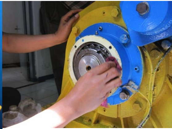
Figure 25: Inspection of a sidewall mounted bearing of a T15 crossflow turbine.
