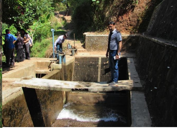
Figure 96: Filling of the forebay tank.
