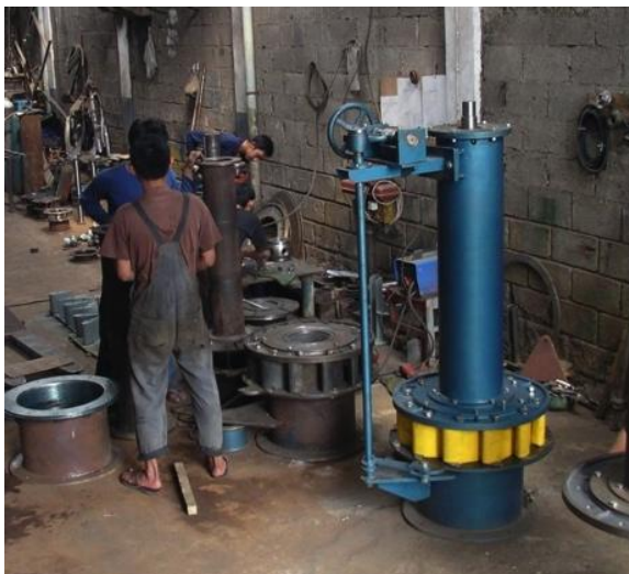
Figure 28: Open flume propeller turbines under construction. The guide vane (yellow) and vertical adjusting mechanism is visible to the side of the runner shaft casing.
