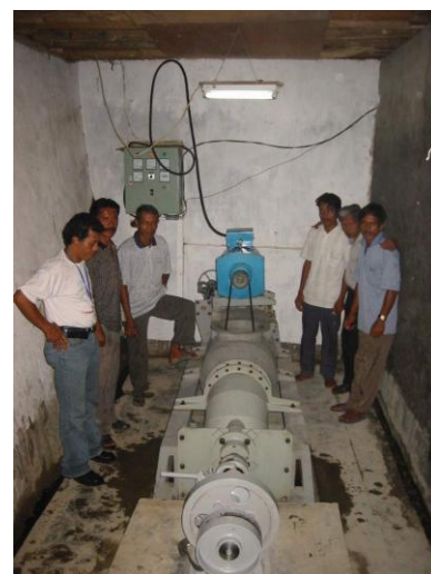
Figure 62: Locally manufactured propeller turbine.
