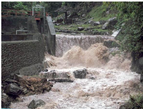
Figure 11: Picture of flood flow at weir
