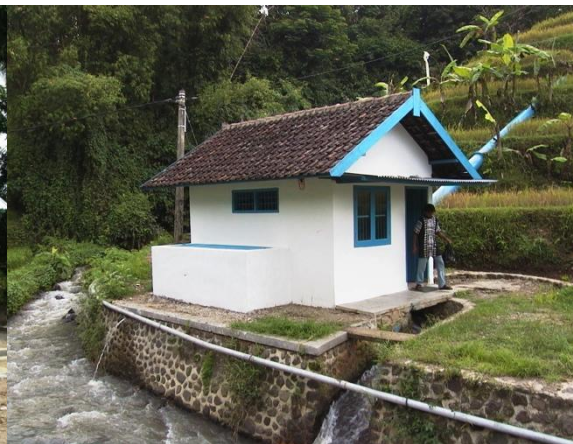
Figure 52: Typical powerhouse and tailrace situated alongside an irrigation channel.
