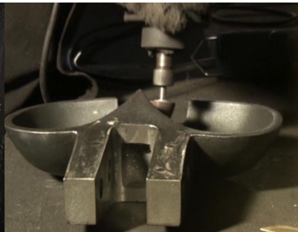
Figure 31: Final polishing of a pelton bucket after rebuilding work.
