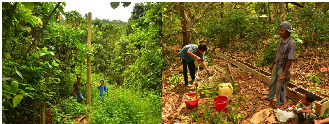
Figure 79: Locally cast concrete cable pole being erected.
