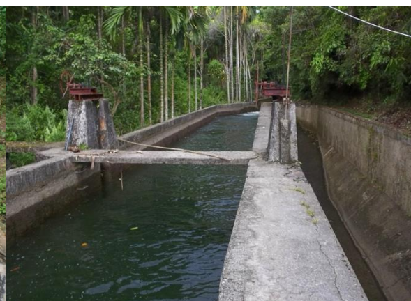
Figure 26: Example of a setup with 2 parallel settling basins enabling scouring to take place without the need to shut down the plant.
