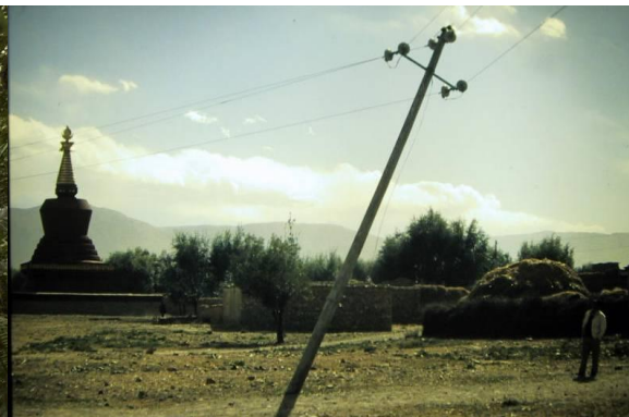
Figure 53: Leaning cable pole posing a safety threat.
