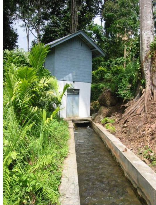
Figure 54: Double level powerhouse and tailrace. As flood protection the powerhouse is positioned well away from the river.
