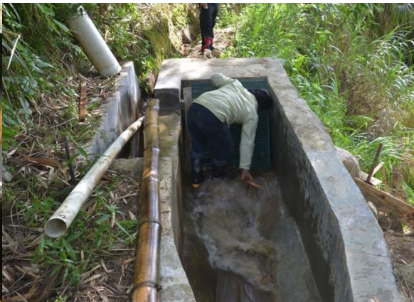
Figure 92: Flushing the forebay tank.
