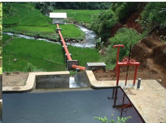
Figure 102: Water in the forebay must be maintained at the full level during operation.
