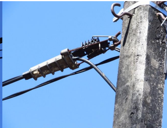
Figure 84: Standardized ABC twisted cable tensioner.
