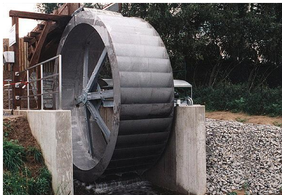
Figure 1: Modern day steel overshot waterwheel for electricity generation.
