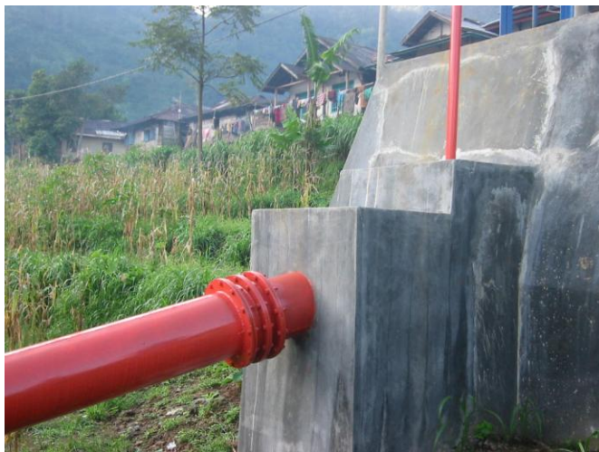
Figure 47: Expansion joint fitted correctly immediately after an anchor block.
