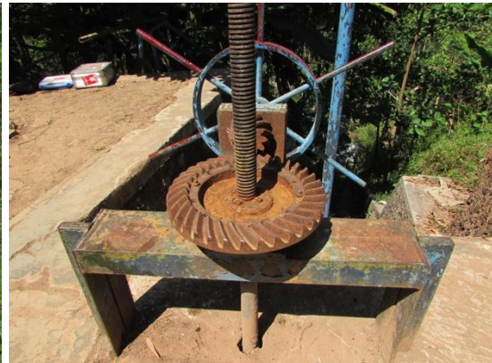
Figure 108: The penstock shut off valve is commonly positioned in the forebay tank.
