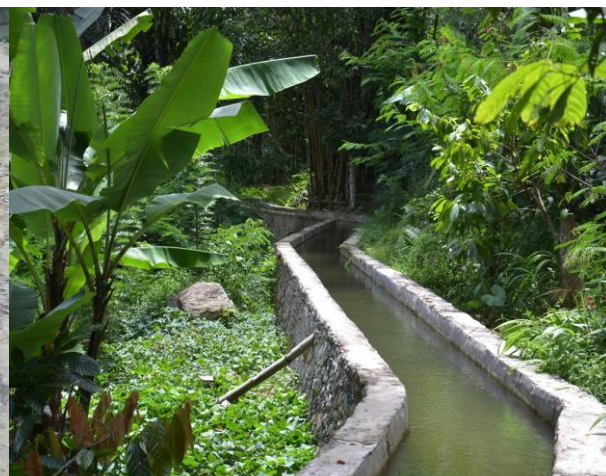
Figure 16: Properly maintained and functioning above ground stone masonry headrace channel.
