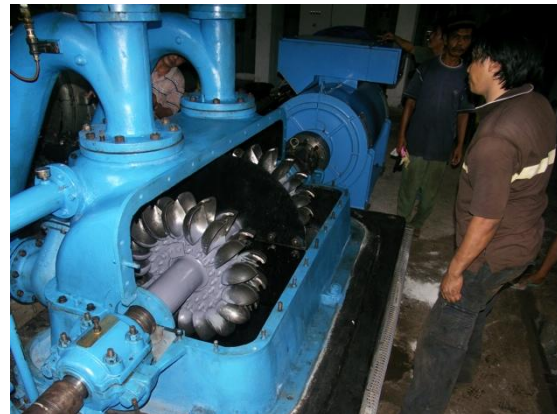
Figure 58: Pelton turbine undergoing maintenance.
