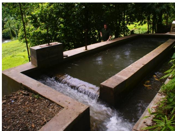
Figure 99: Water spilling over the front of the trash rack. This design facilitates a degree of self-cleaning as the water passes over the trash rack taking floating debris with it.
