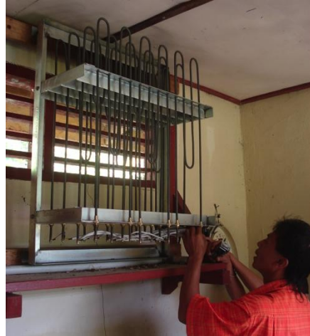
Figure 90: Periodic inspection of the ballast load and cables is important.
