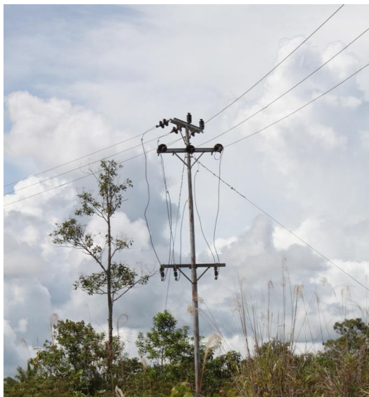
Figure 77: Typical transmission line using traditional un-insulated cables.
