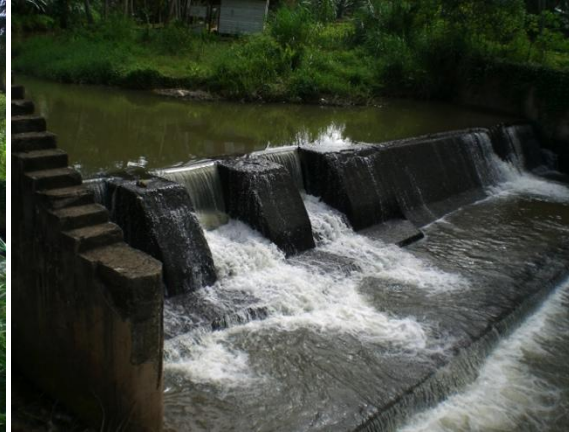
Figure 24: Combined concrete and stop log weir construction.
