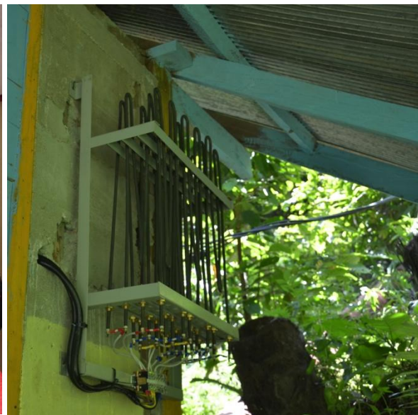
Figure 47: Externally installed air ballast.
