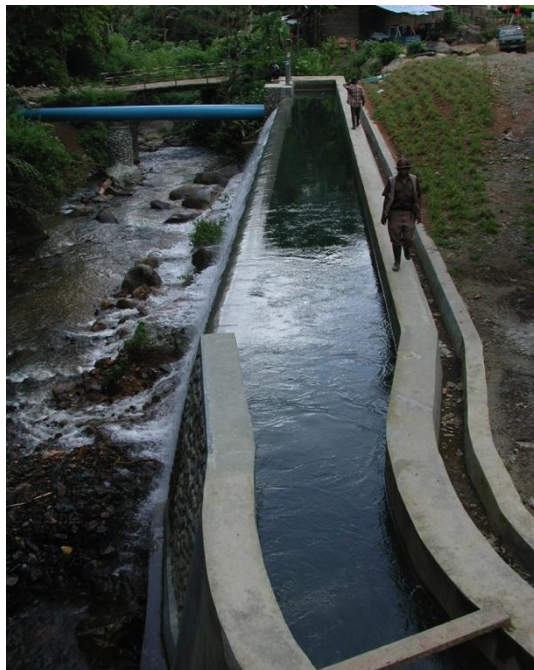
Figure 27: Conventional settling basin with a spillway over its full length. A pipe bridge exit to leading to headrace is visible.
