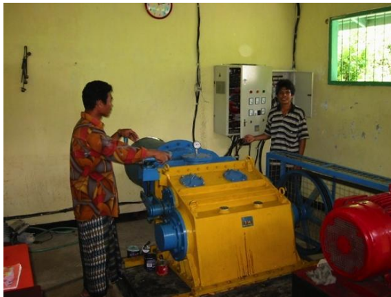
Figure 75: Typical manually controlled cross flow turbine governed by an electronic load controller (ELC).
