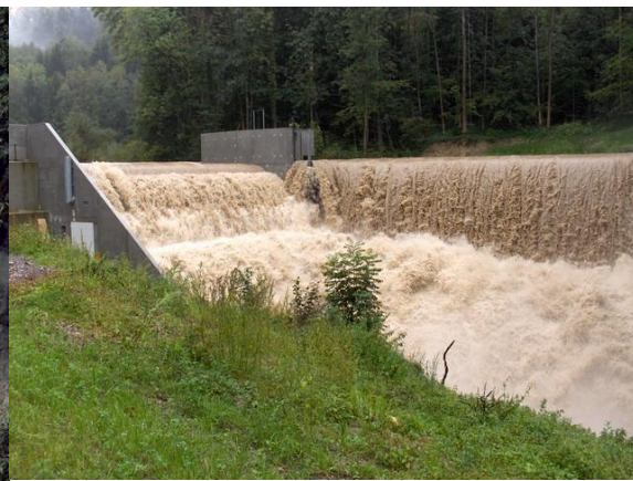
Figure 12: High flow going over weir
